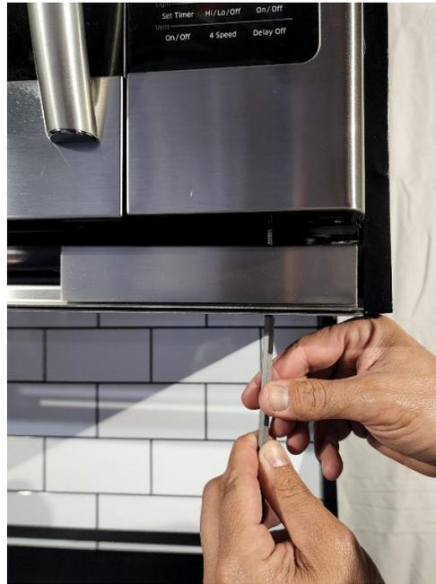
**Step #5:** Once both adapters are installed, and flush with outside edges of microwave unit frame tighten both screws until seated firmly. You do not need to over tighten, just make sure to tighten the screws firmly.
