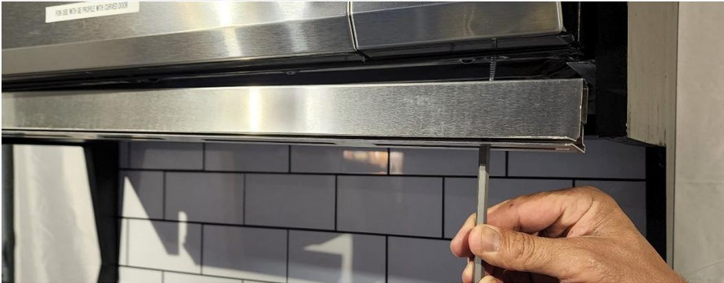
**Step #5:** Once that is completed, and the brackets are centered, tighten center screw until seated firmly. Now move to the balance of the other screws and tighten until firmly snug. You do not need to over tighten, just make sure to tighten the screws firmly.
